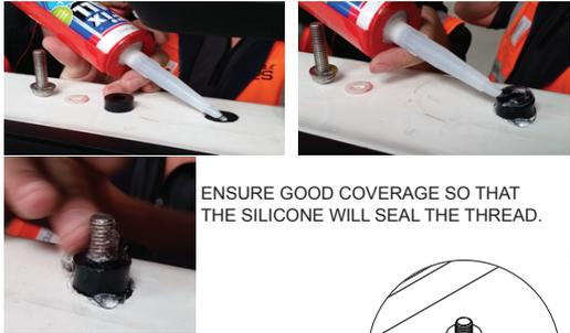
ENSURE GOOD COVERAGE SO THAT THE SILICONE WILL SEAL THE THREAD.
