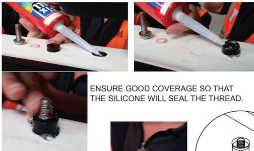
ENSURE GOOD COVERAGE SO THAT THE SILICONE WILL SEAL THE THREAD.
